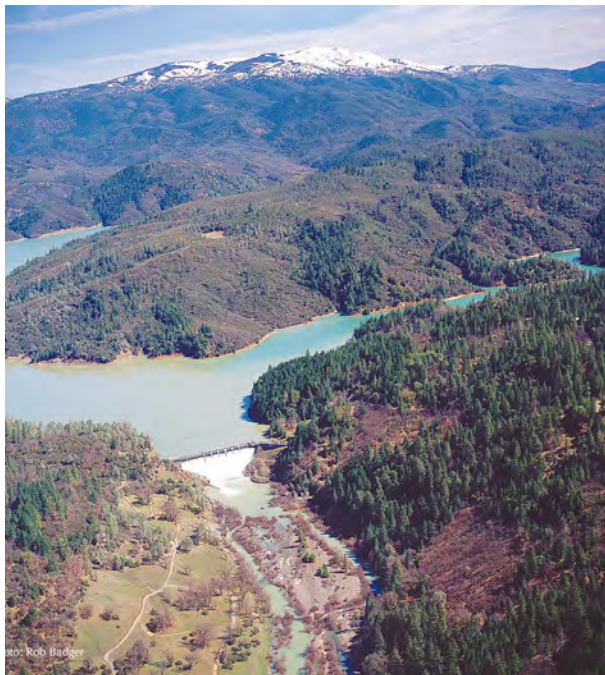
Scott Dam, one of two Eel River dams. Scott Dam impounds the river to form Lake Pillsbury Reservoir. Ask FERC to initiate license surrender for Eel River Dams to begin dam removal. Photo credit: Rob Badger.
